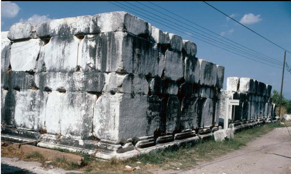
Exterior looking northeast
