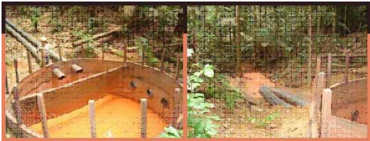
Figure 3: Sediment control structure for a bauxite mine (MRN) in Brazil. Water energy dissipation tank (left) and discharge point (right)
