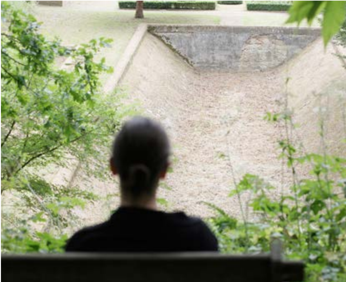
"Dry the pool, dry concrete, brown edged"
