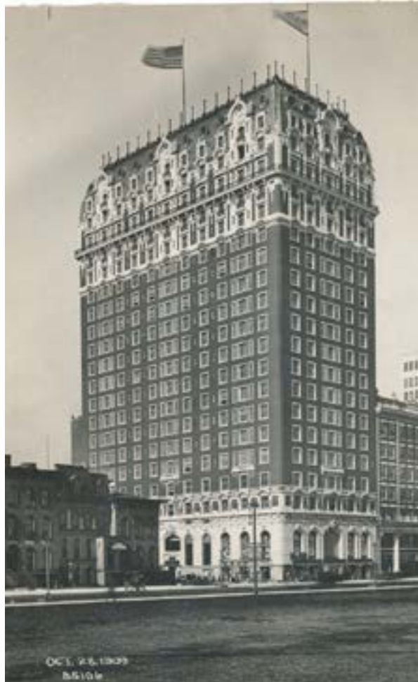
Blackstone Building, Chicago 1909
