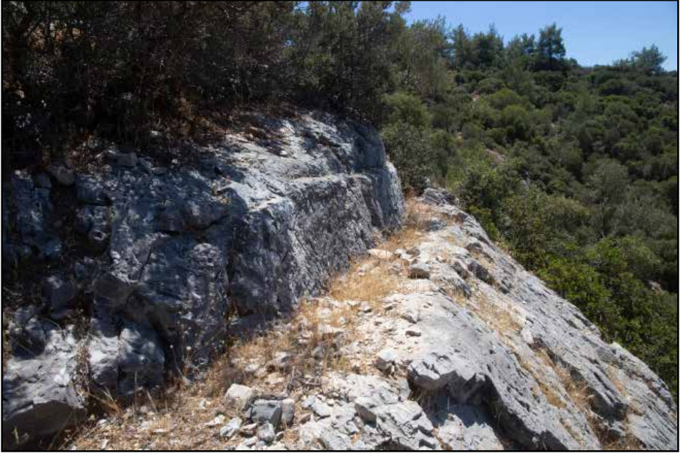
Figure 10: View from northwest of channel of aqueduct
